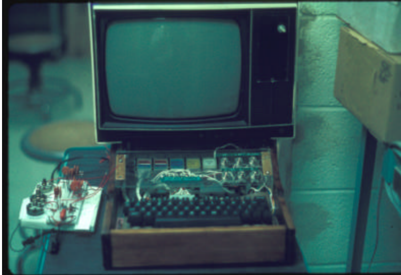
1973 – Sol Libes & students build terminal/serial interface using old TV & interface it to IBM 360 computer & ARAPNET via Rutgers University
